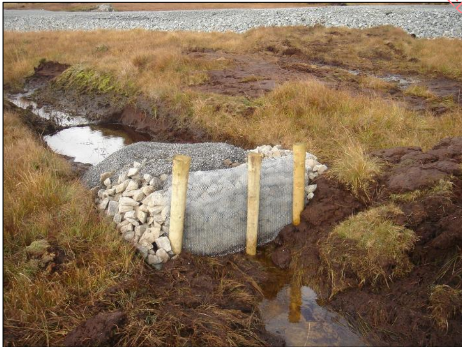
Figure 5-3 – Typical Check Dam
