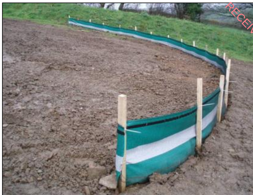
Figure 5-2 – Typical Terrastop Silt Fence
