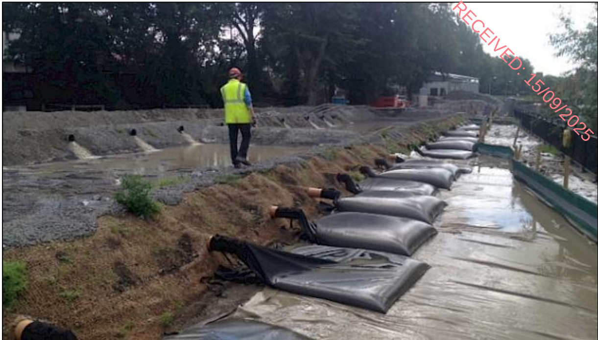
Figure 5-6 – Typical Silt Bag Installation
